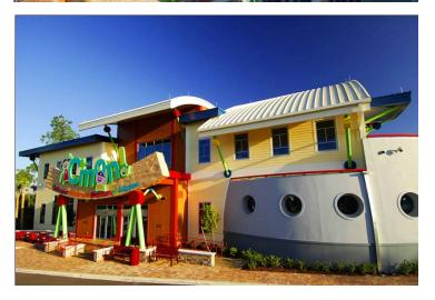
"The concave and convex curves of the roof (design) made this a particularly challenging project," recalls Scott Otey, Vice President of West Coast FI Enterprises, Inc. commercial roofing, "Every flashing detail had to be carefully fabricated."
