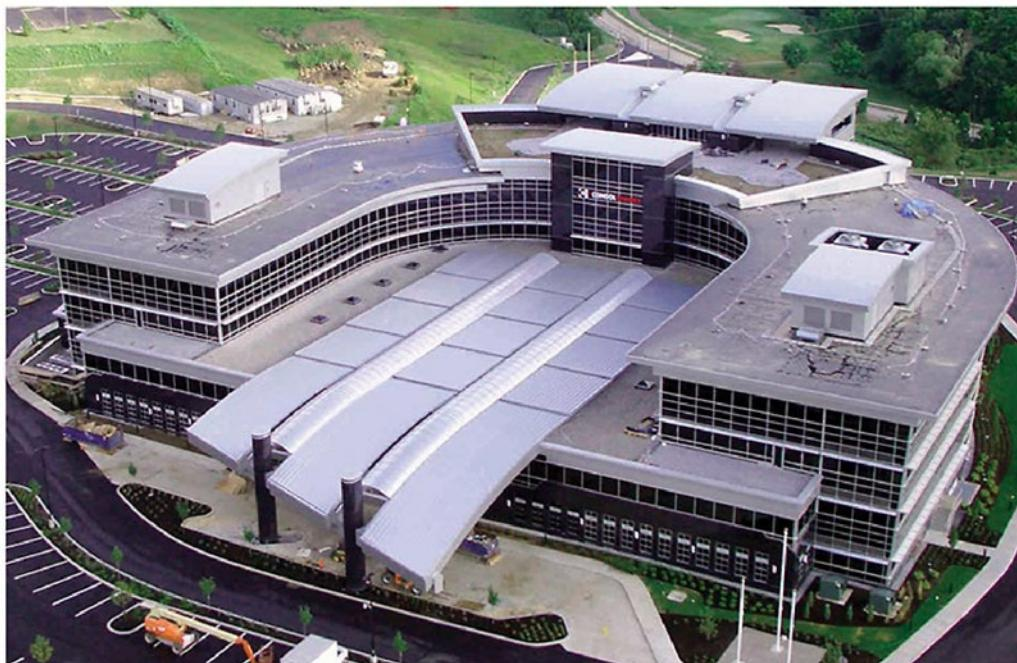
were sloped and concave, convex and flat in shape," Viehman explains. "And the upper and lower fascias were at different radii in the curved areas, all of which would create problems for fabrication and installation. We also determined the substrate we were attaching to was not square and plumb, which further exacerbated the entire process. Realizing all of this, we knew we had to plan the job properly before going into mass production of the panels."
