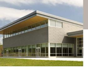
between various cladding materials. In many face-sealed wall systems, caulking is commonly used to create these seals, requiring perfect installation. In addition, no caulking is permanent. It degrades over time, usually as soon as five to ten years. Caulking can stain, collect dirt, and is costly because it necessitates close monitoring and maintenance.
